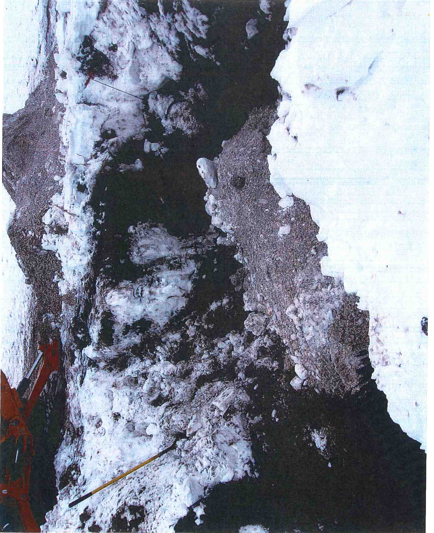
PLACING ROCK AROUND 15" HOPE
